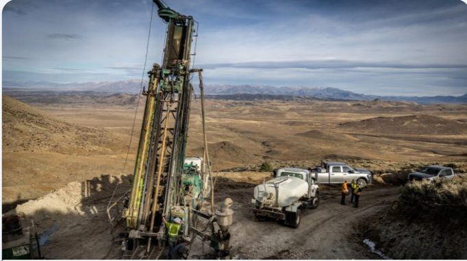
South Carlin Complex 2 Nevada, USA
