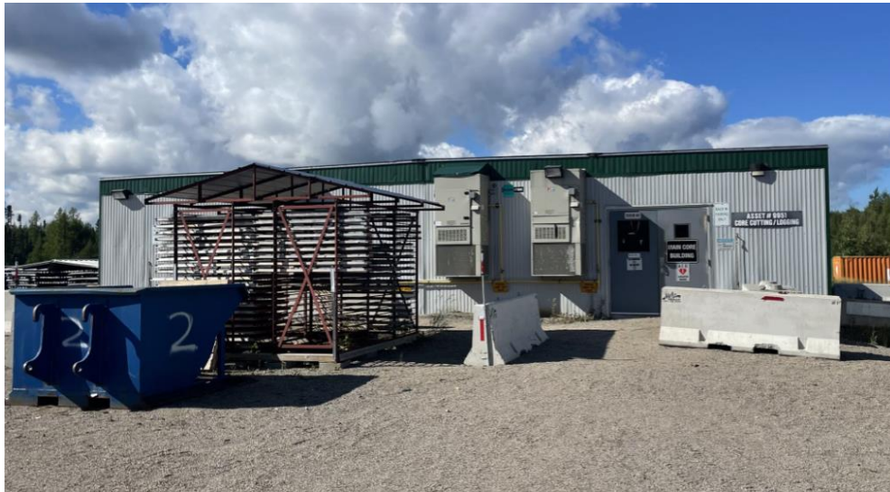
Figure 10.3 – Exploration Core Shack
