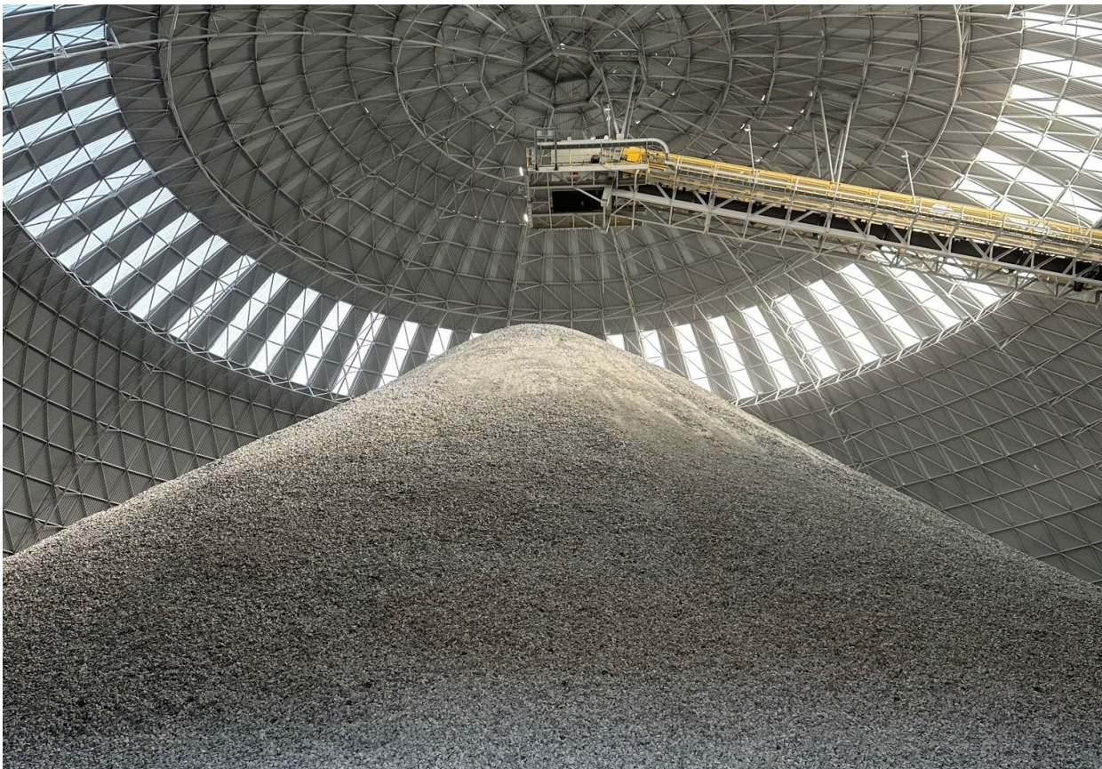
Crushed ore storage dome.
