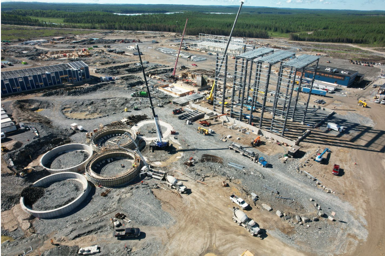
Figure 1 - Concrete foundations for leach tanks (foreground left), steel structure for west end process plant (foreground right), administration building (back right), truck shop (back centre), power plant (back left)
