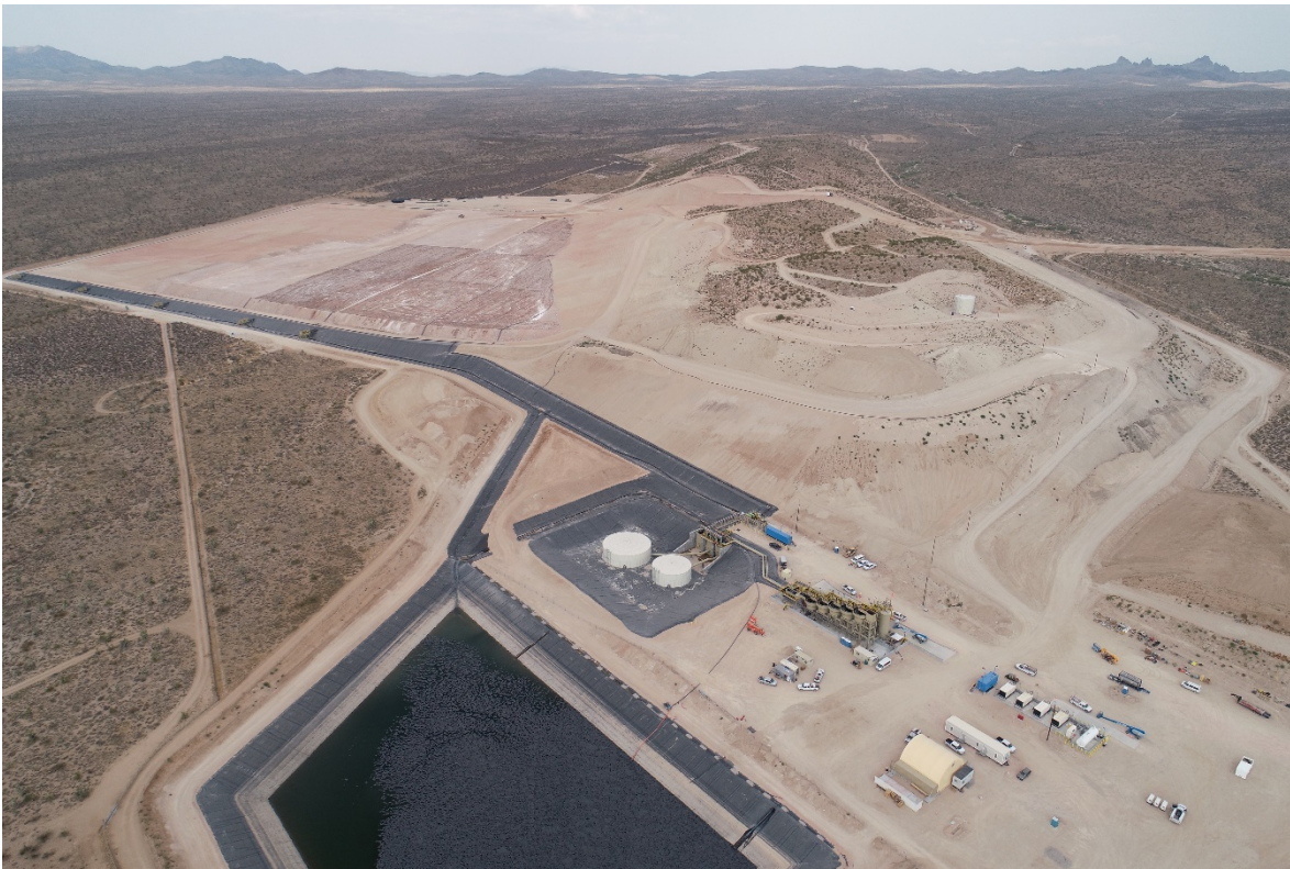
Figure 1 - Castle Mountain Phase 1 heap leach pad (background) and processing facility (foreground)
