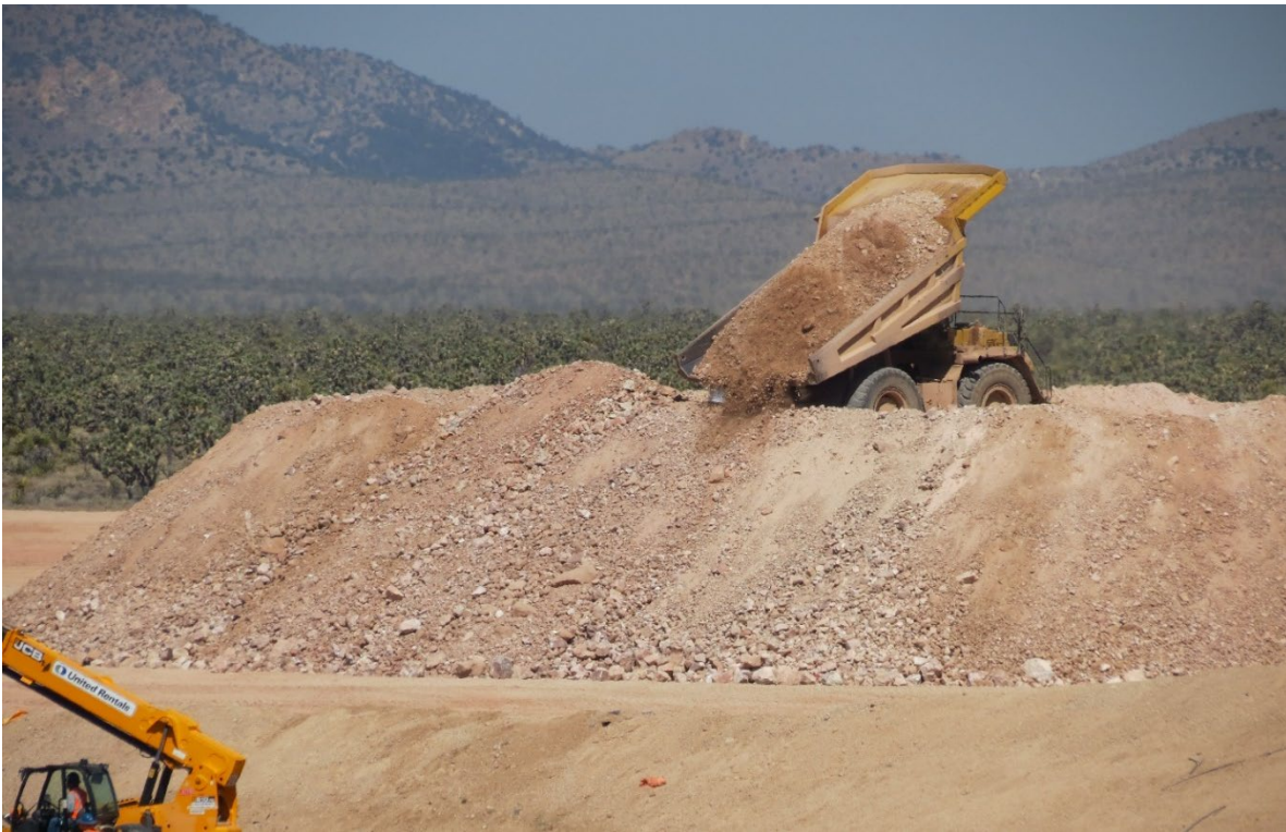
Figure 3 - Stacking ore on leach pad
