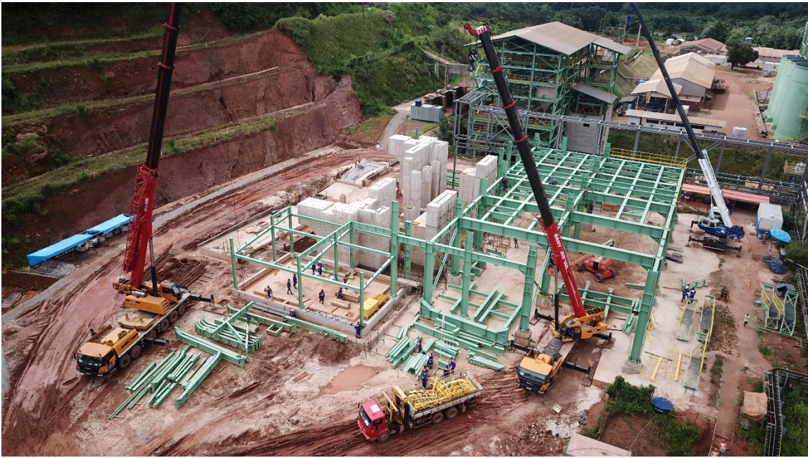
Foundations and framework for new SAG and ball mills
