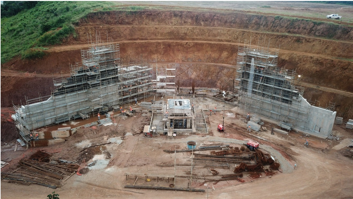
Foundations and framework for crusher
