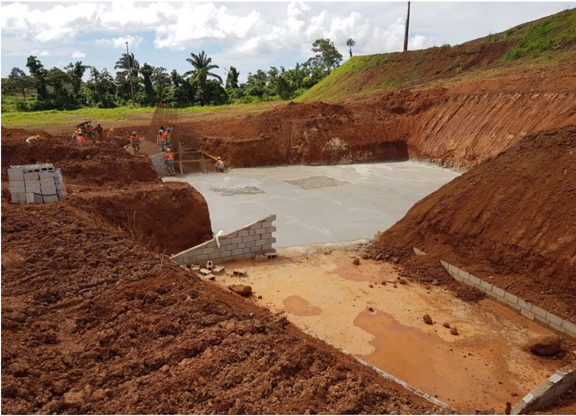
Stockpile area: bulk earthworks complete, concrete works underway
