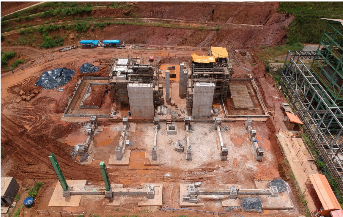
Concrete foundations and pedestals in place for new SAG and ball mills
