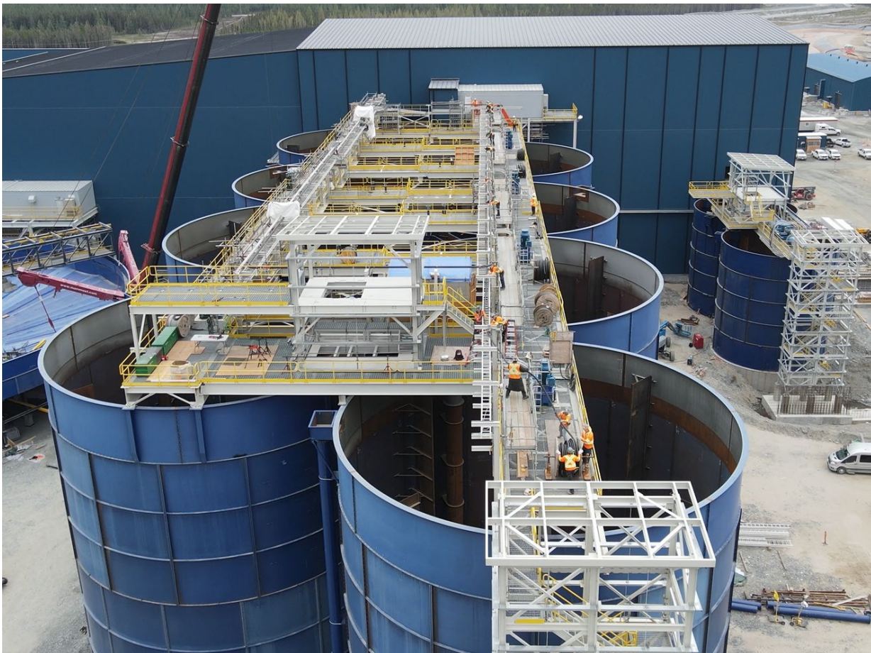
Cable pulls on leach tanks
