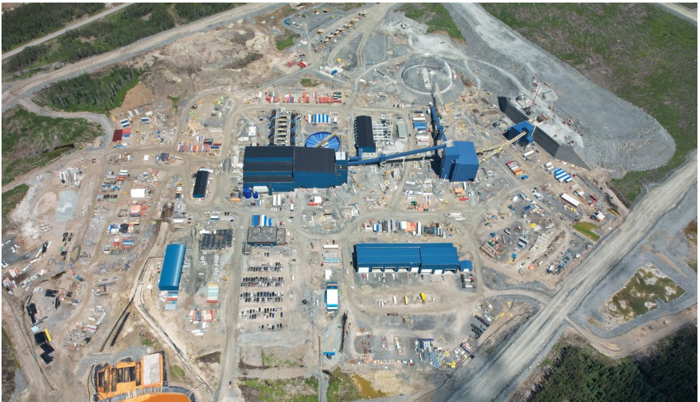
Plant site overview – July 21
