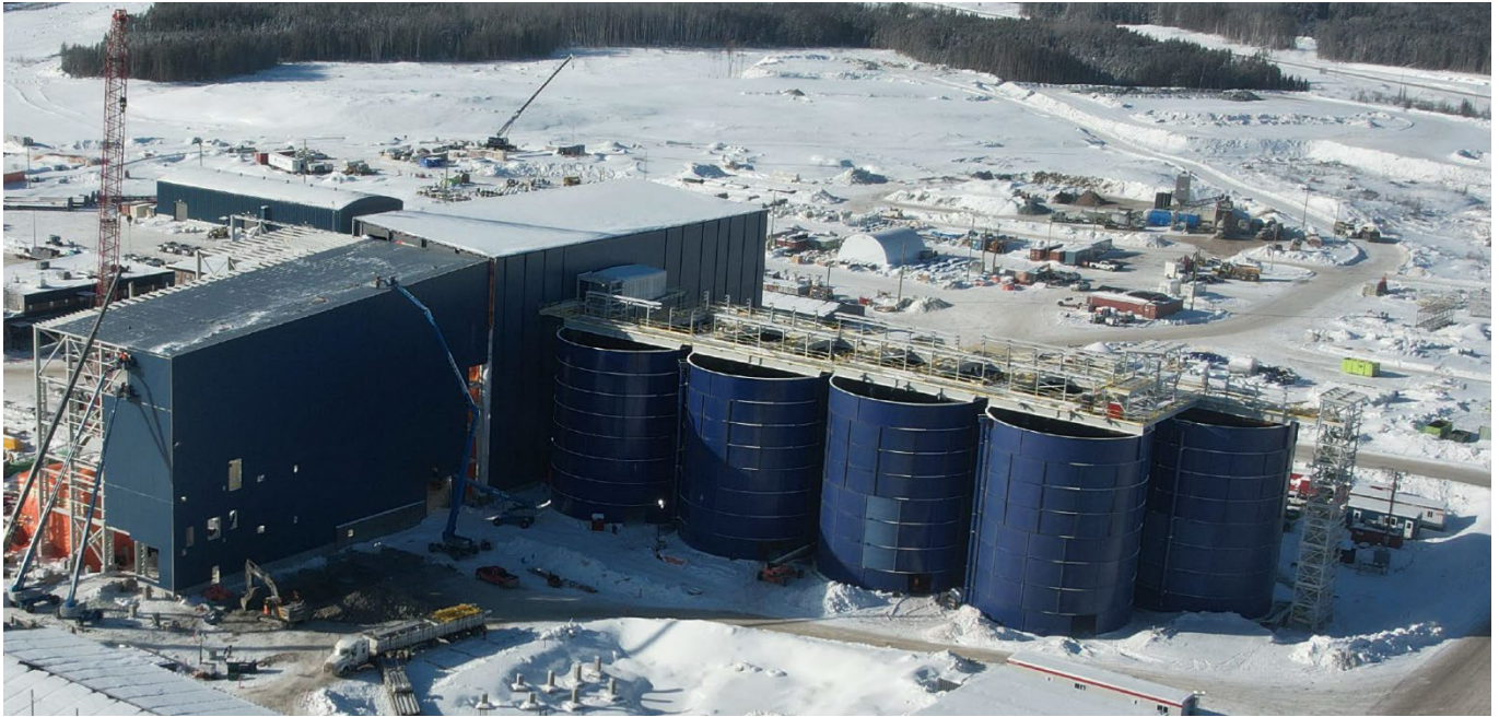
Leach tanks and process plant.
