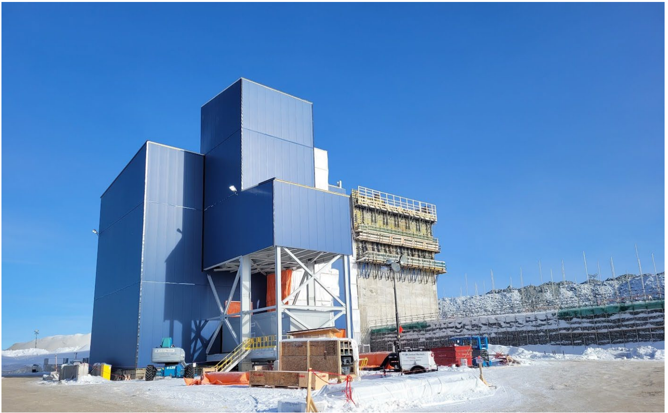
Primary (right) and secondary (left) crushers – exterior.
