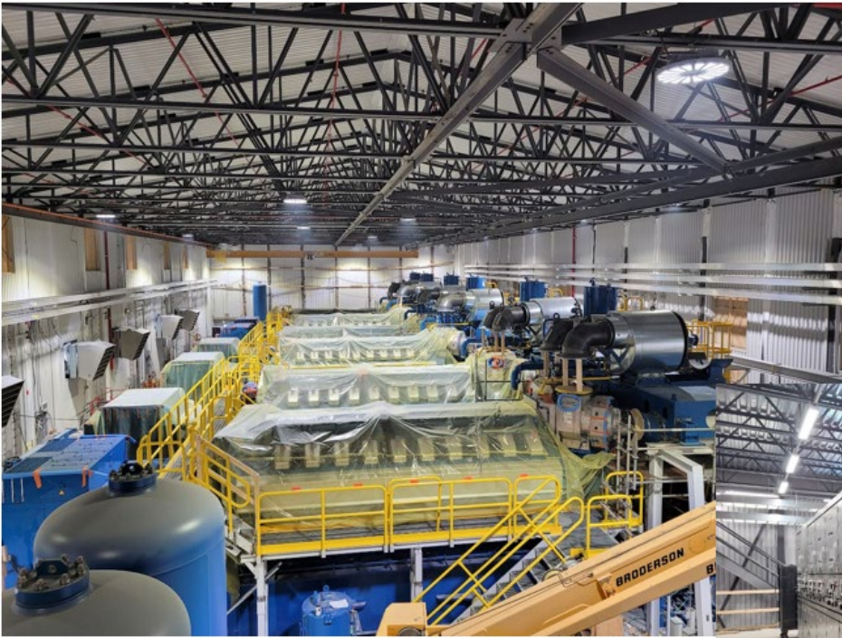
Power plant – interior.
