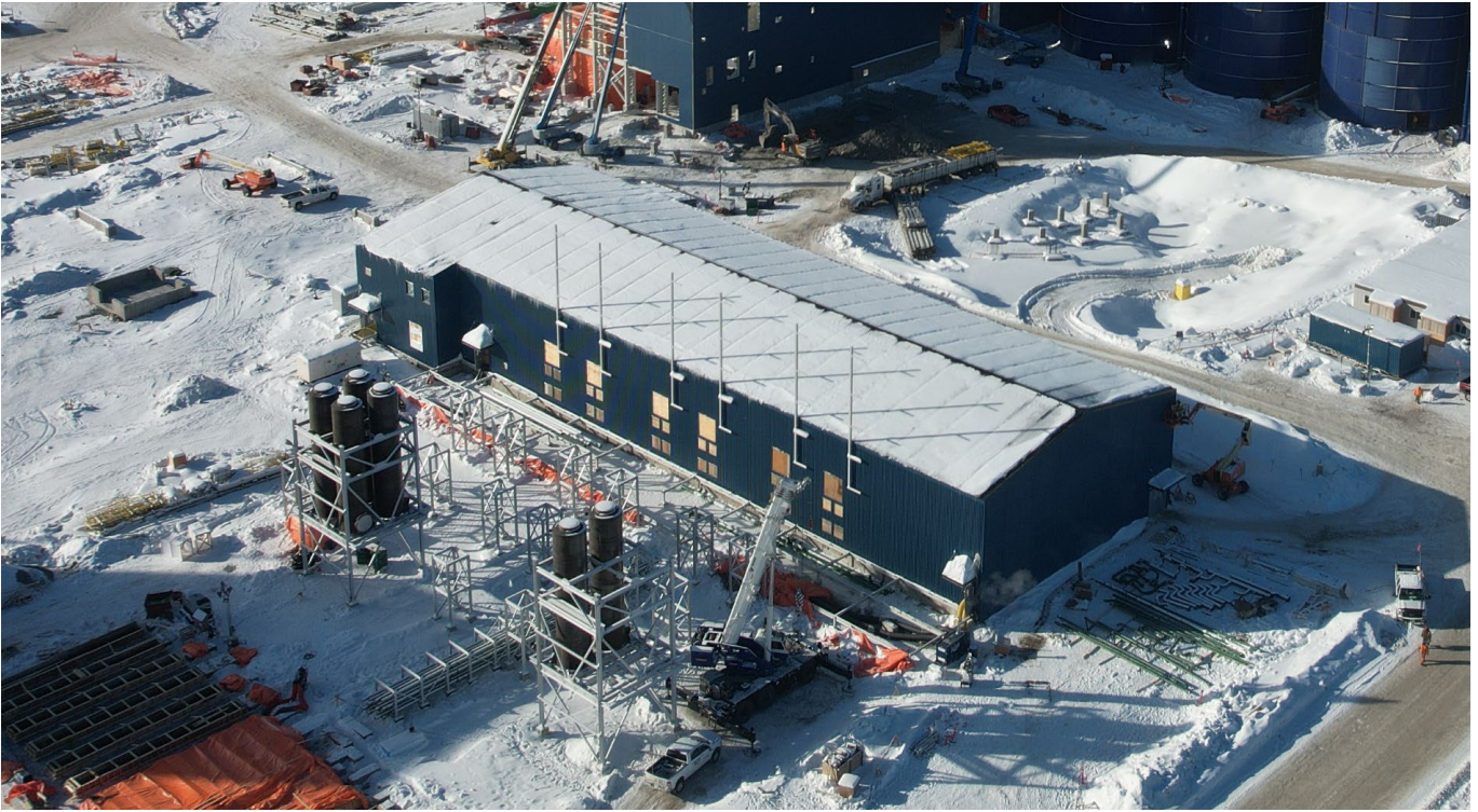
Power plant – exterior.
