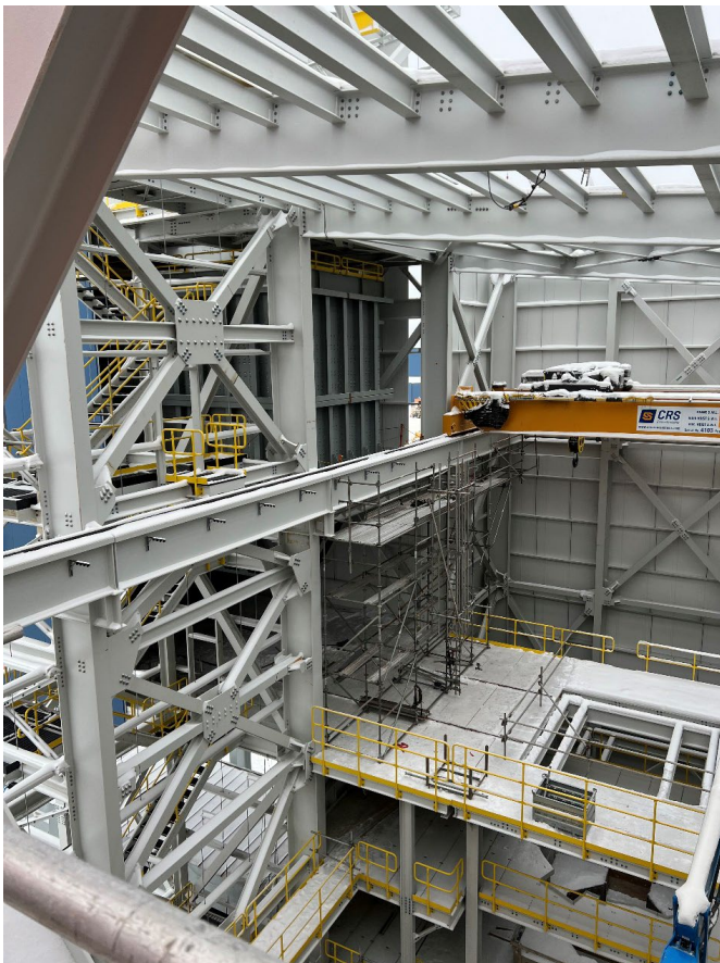
Secondary crusher – interior.
