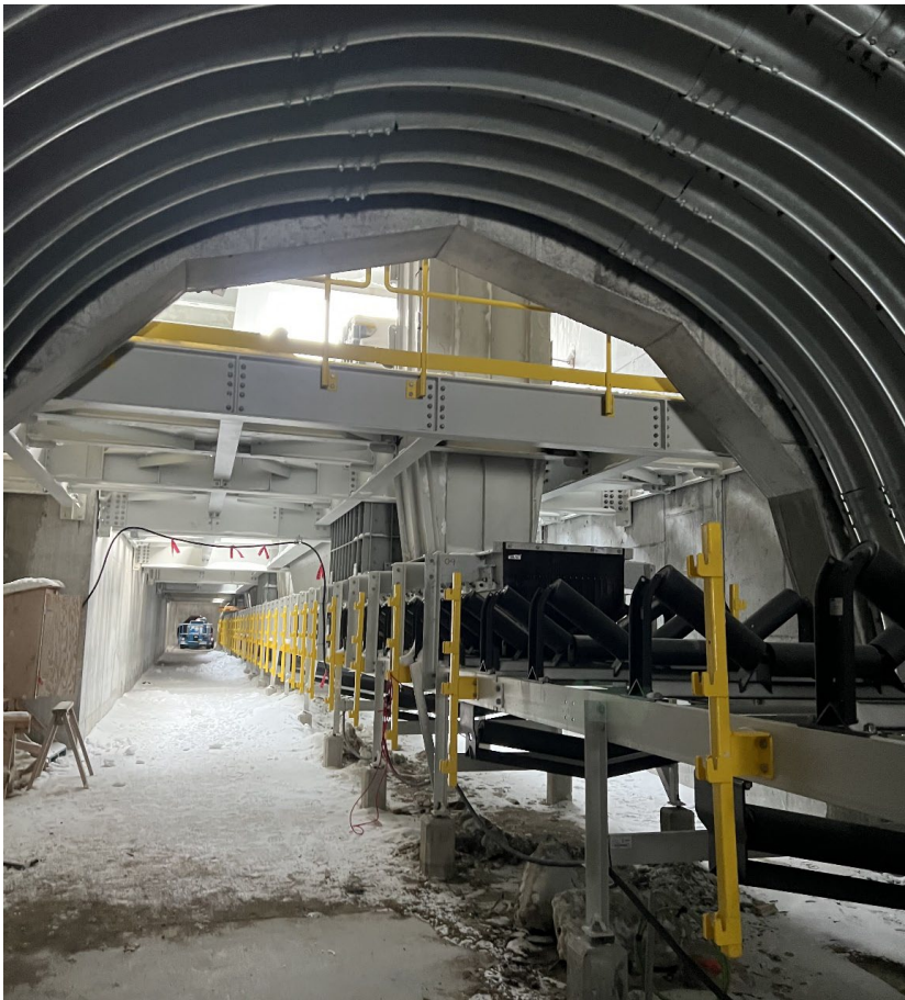
Reclaim tunnel with conveyer and chute.
