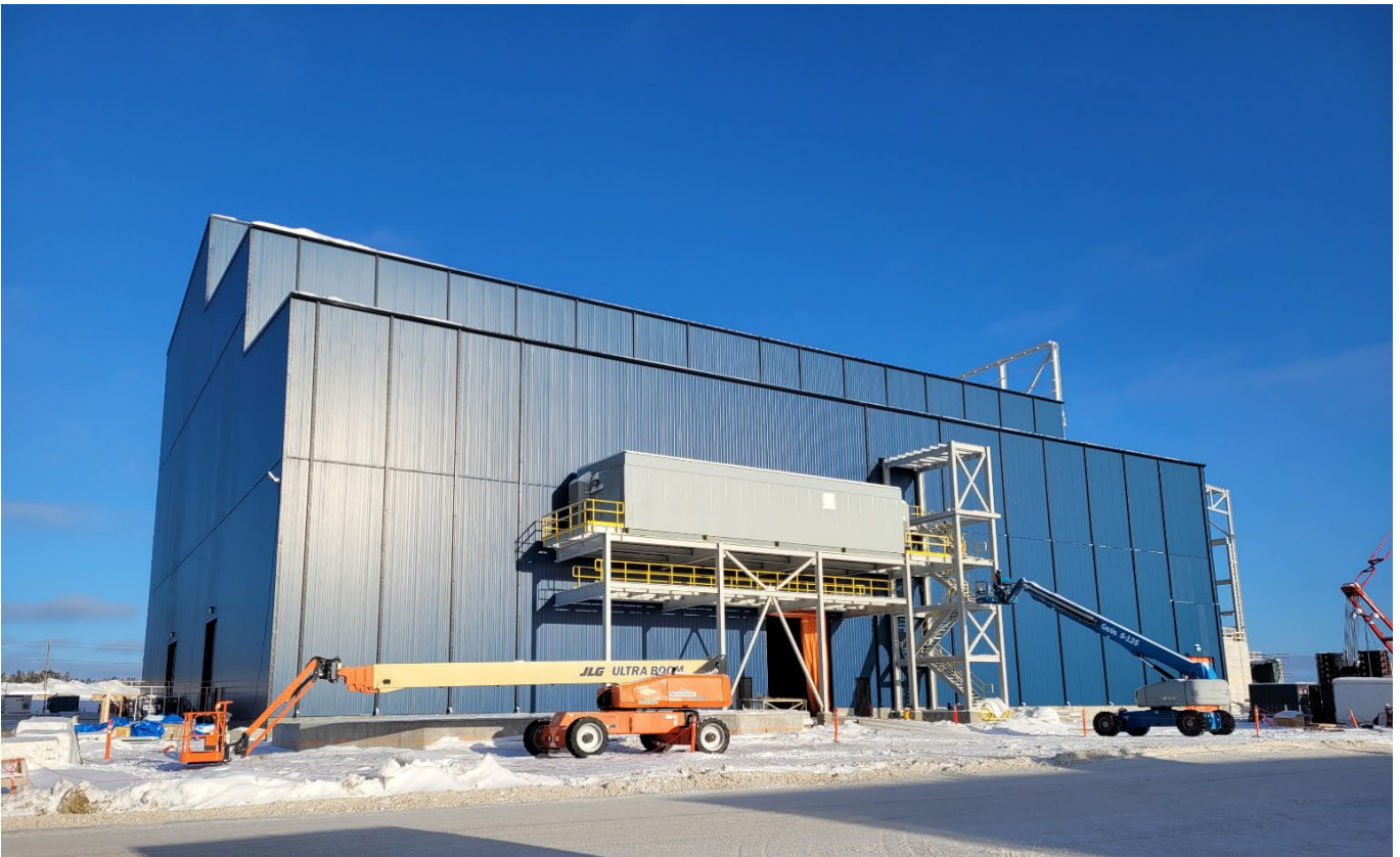
West end process plant with e-room.
