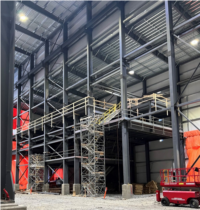
West end process plant – interior.
