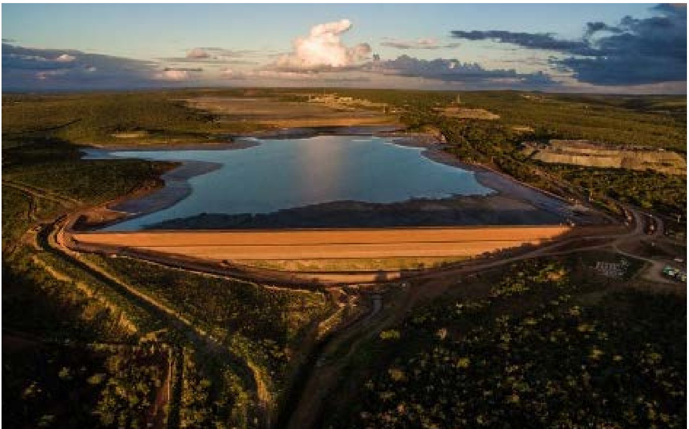
Fazenda – Operating facility
